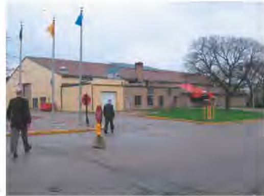
View Looking North East
