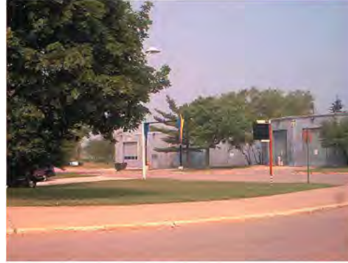
View Looking North East
